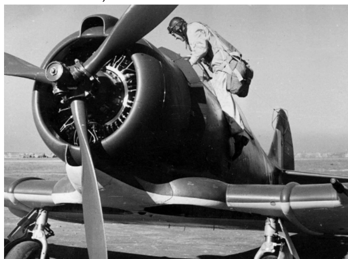
Above: Ken Frewin boards A46-1 prior to its first flight. Notice the early style of engine cowling with the oil cooler air intake below the circle of the cowling. This style was only fitted to the first two Boomerangs. Also visible is a protective wire cage around the top of the fin, perhaps to protect the rudder from fouling if the antenna wire broke.
