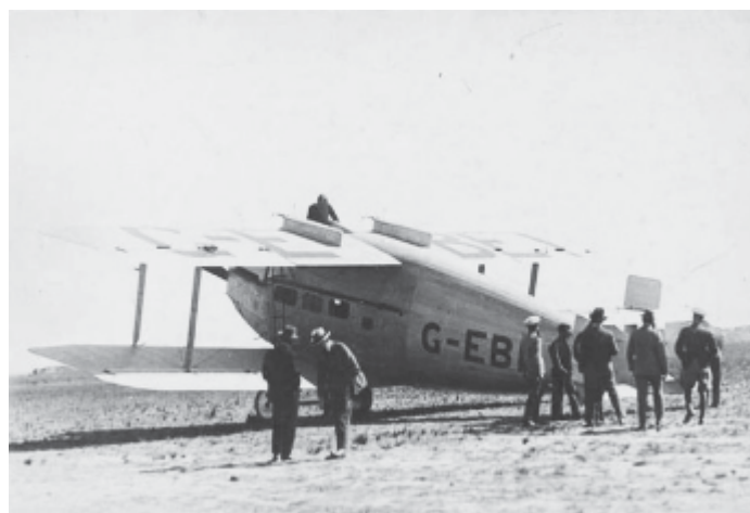
Above: Another view of the Vulcan, possibly at Longreach during the flight testing. Fuel tanks mounted above the upper wing are obvious. Photo: NLA
